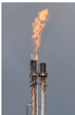
Figure 12, Refinery flare tower
